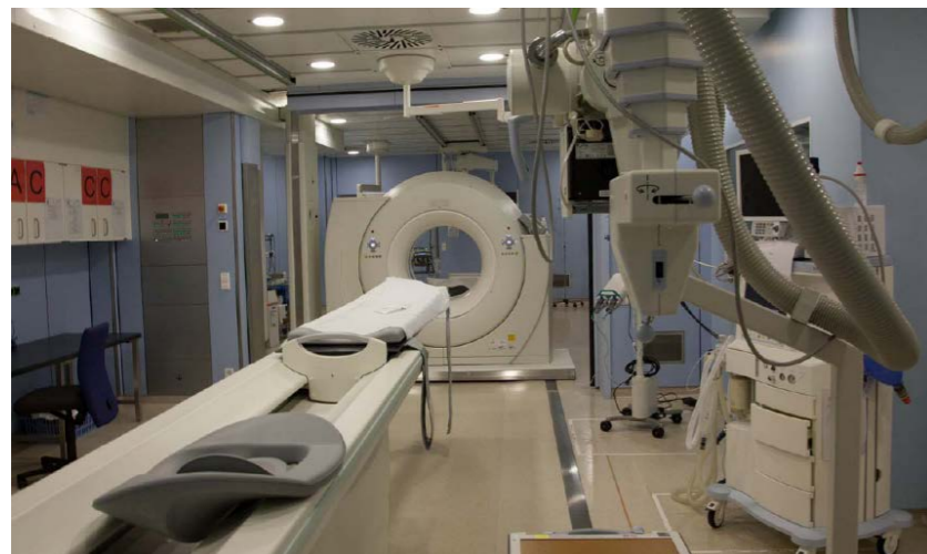
View of our trauma room with a sliding gantry solution. In the back, the sliding gantry is in its normal position in the standard CT examination room. The CT suite and the trauma room are separated by a sliding X-ray-proof (background) door. If CT is required for a trauma patient, the door opens and the gantry slides over. The patient is scanned without the need for any further relocation.
